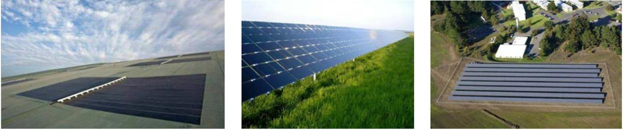
**Figure 4. Thin-film solar panels installed on (left) solar energy cover and (middle/right) fixed-tilt mounting system. Photos from (left) Republic Services, NREL 23817, (middle) Beck Energy, NREL 14726, and (right) U.S. Coast Guard Petaluma Site, NREL 17395**
