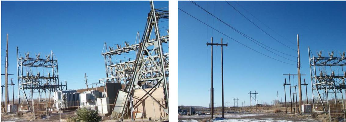
**Figure 10. Electrical tie-in point of 24-kV and 115-kV lines for the PV system at the Chino Mine. Photos by Kosol Kiatreungwattana and Lars Lisell, NREL**
